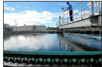
12 Mile Creek Water Treatment Plant (Not in Marvin and Administered by Union County Public Works)
