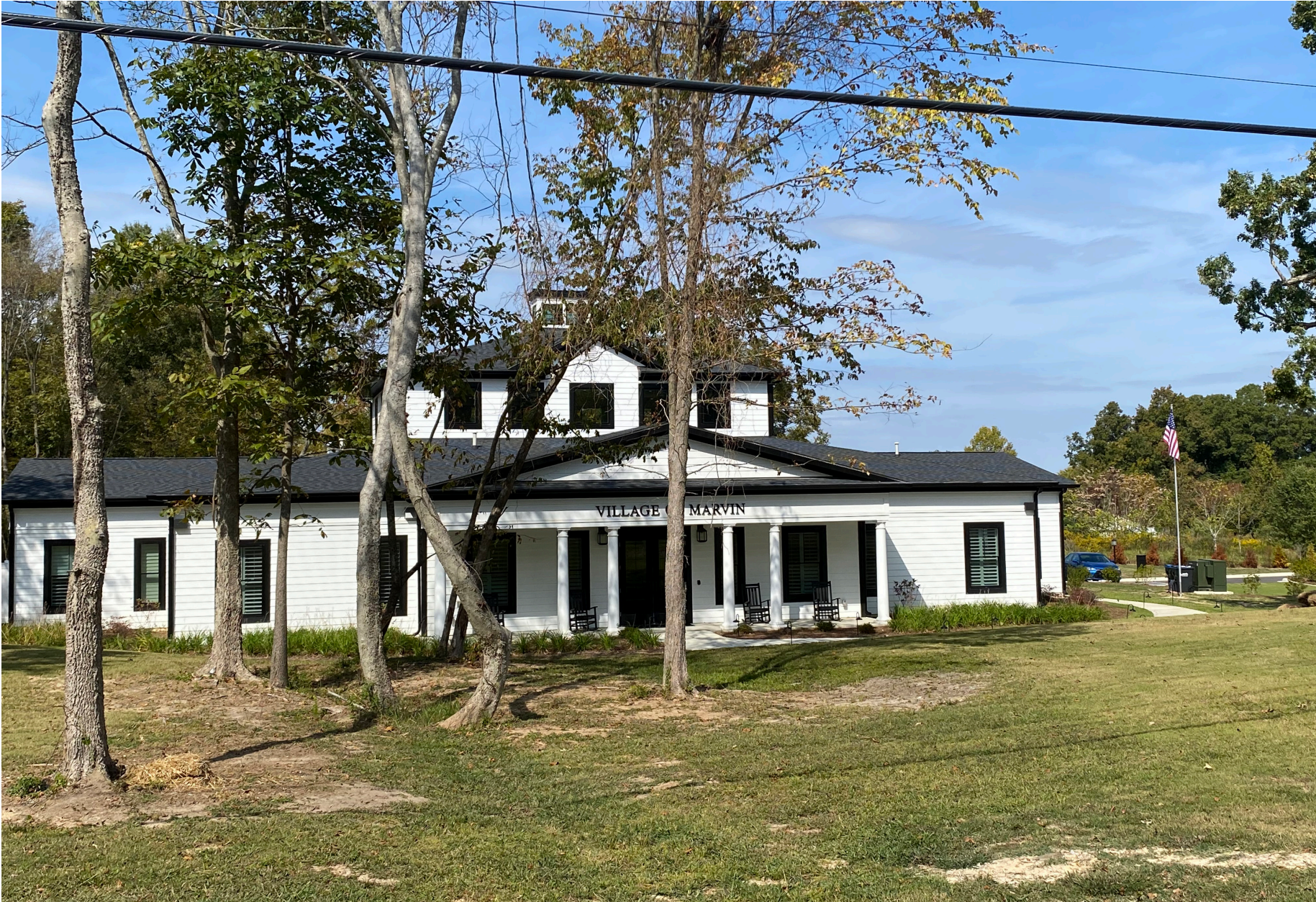
View of Village Hall from New Town Road / McAdams
